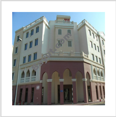
England Exterior View 4
