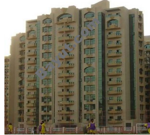
Al Rashidiya Tower exterior1
