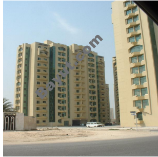
Al Rashidiya Tower exterior
