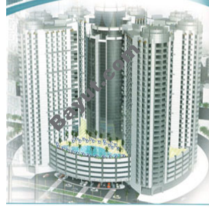
Falcon Tower Exterior
