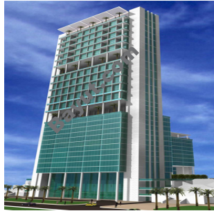
Liberty House Exterior View 1
