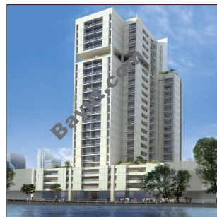
Clayton Residency Exterior
