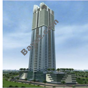
Abjar Tower Exterior View 2
