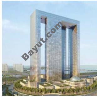
Dubai Pearl Exterior View
