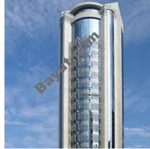
Al Attar Business Tower Exterior View 3
