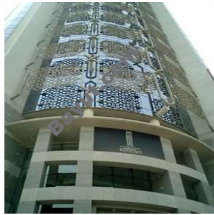
Al Attar Business Tower Exterior View 2
