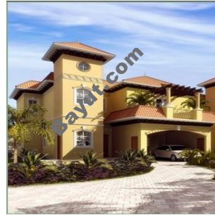
Gallery Villas Exterior View
