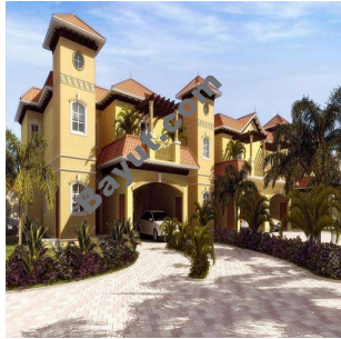
Gallery Villas Exterior View 2
