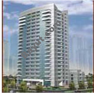
Marina Diamond 5 Exterior View
