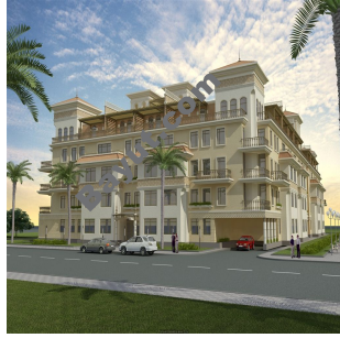
Astoria Residence Exterior View
