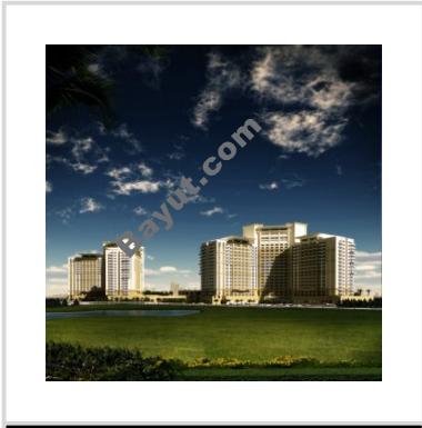
Jumeirah Heights (Village Centre) Exterior View
