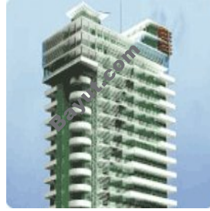
Rufi Golf Green Tower Exterior View 2
