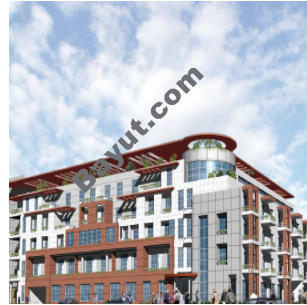
Elements Exterior View 2
