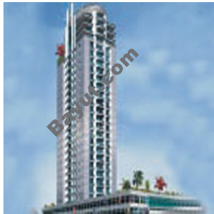
Marina Wharf 1 Exterior View 3
